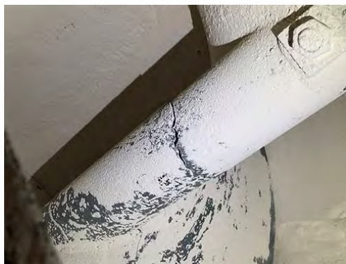
Existing Center Pipe of Screw Failed and Shut Down the Process
