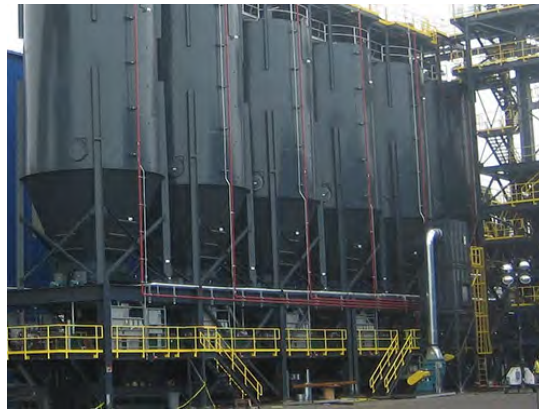
Large Silos Store Coal-Based Bulk Materials
