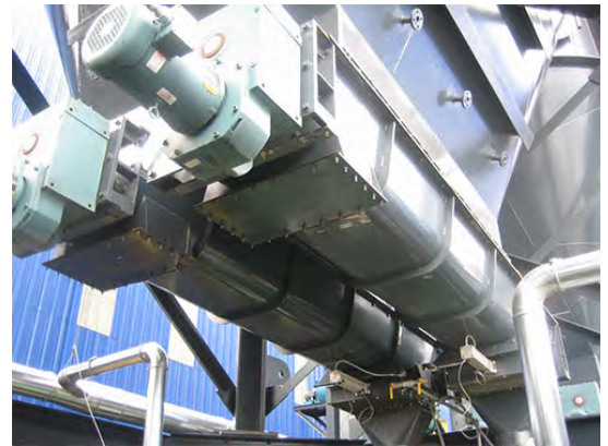
Twin Mass Flow Screw Feeders Accurately Meter Bulk Materials
