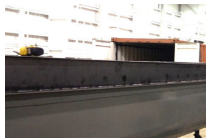
Welded Trough Channel Extensions at Soil Remediation Plant Allow Air to Cool Soil from Dryer
