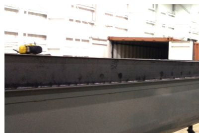
Welded Trough Channel Extensions at Soil Remediation Plant Allow Air to Cool Soil from Dryer
