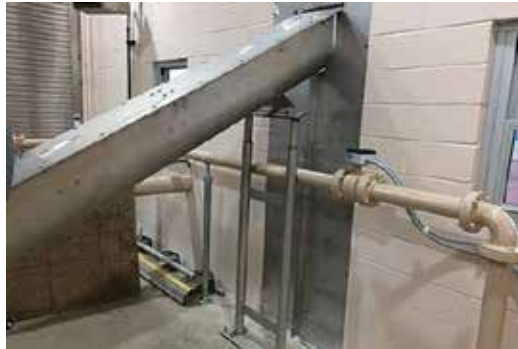
Vertical Height of Pipe Support is Easily Adjusted and Welded in Place
