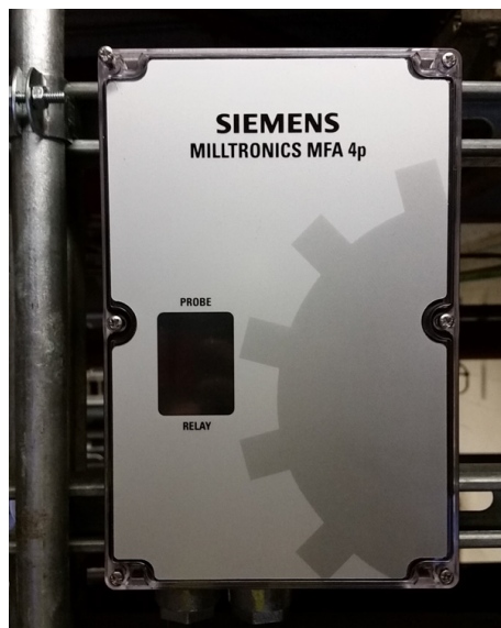
Milltronics MFA 4p Controller Can be Mounted Near Equipment or as Far Away as 200-Feet in Non-Hazardous Environments
