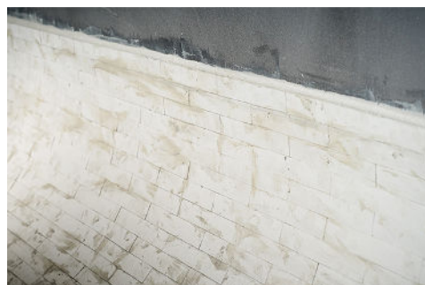
Grout Layer Between Trough and Liner achieves Seamless Internal Surface
