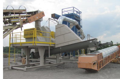
Screw Conveyor Transfers Pulverized Limestone from Mill to Belt Conveyor
