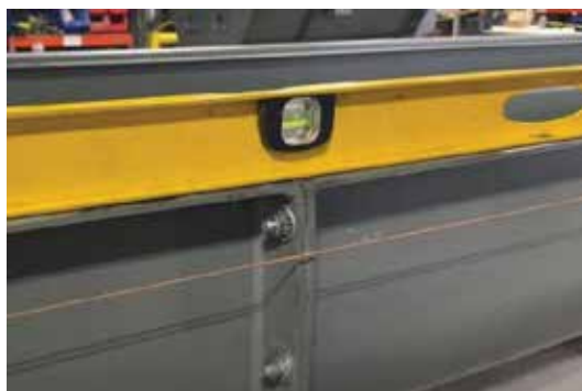
Use Level to Check Levelness at Each Trough Joint – Along Trough Joint
