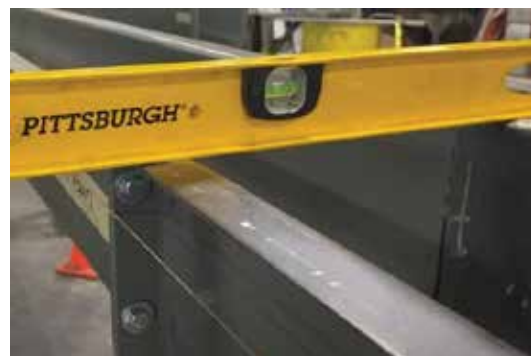
Use Level to Check Levelness at Each Trough Joint – Across Trough Joint
