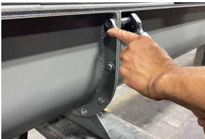
All Fasteners Must be Tightened to Proper Torque Rating
