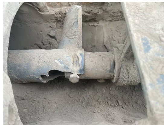
Improper Plug Welds Between Center Pipe of Screw and Internal Collar are Cause of Failure
