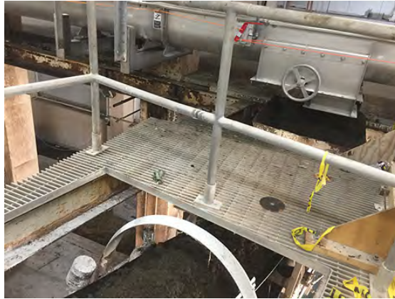
Intermediate Discharge Diverts Dewatered Biosolids to Another Area of the Process
