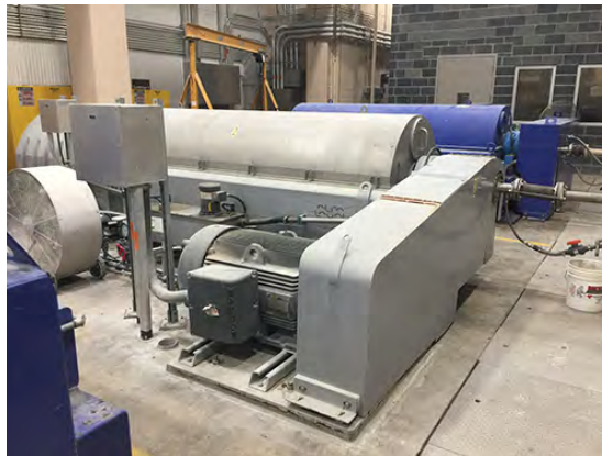
Three Existing Centrifuges Deliver Dewatered Biosolids to the KWS Shaftless Screw Conveyor Load Out System
