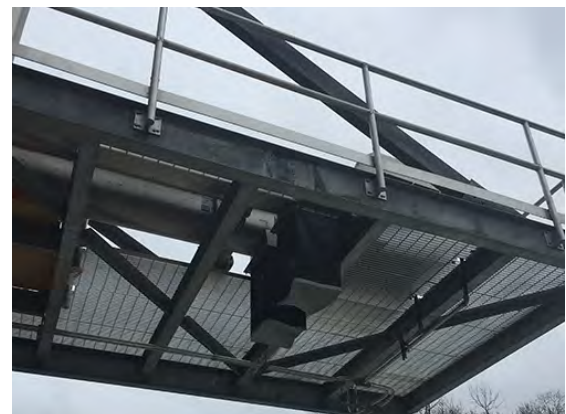
Complete System Redundancy is Provided with Two Load Out Shaftless Screw Conveyors
