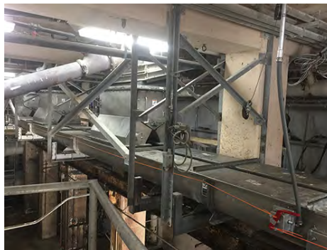
Dewatered Biosolids are Discharged from Three Centrifuges and Diverted into Shaftless Screw Conveyors
