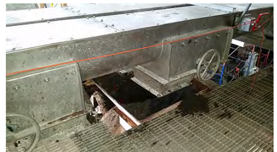
KWS Provided a Curved Slide Gate to Discharge Dewatered Biosolids to Another Area of the Process
