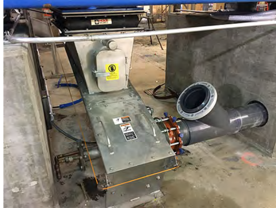
Figure 1: Drain is Located on Non-Carrying Side to Reduce Plugging
