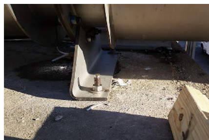
Slotted Anchor Holes are a Standard Feature
