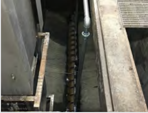
KWS Grit Screw Conveys Grit to a Pump
