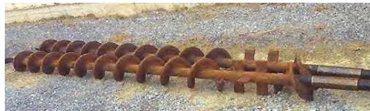
Existing Screws Show a Large Amount of Corrosion and Wear
