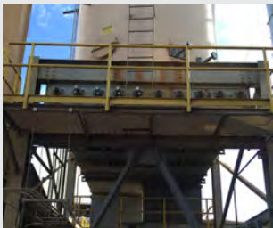
Existing Silo with 12-Screw Live Bottom Feeder
