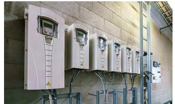
VFDs Can Be Mounted on a Wall Near Equipment
