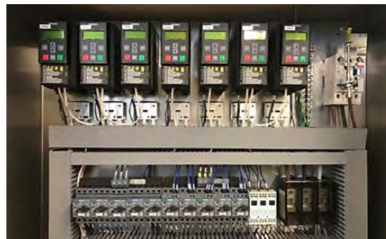
VFDs Can Be Mounted in a Control Panel to Interface with Other Control Systems
