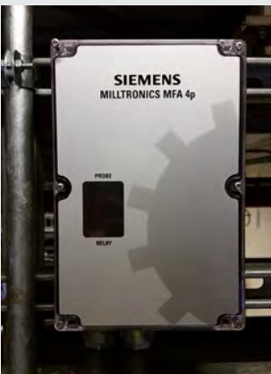
Milltronics MFA 4p Controller Must be Mounted Outside of the Hazardous Environment or Located in an Explosion Proof Enclosure
