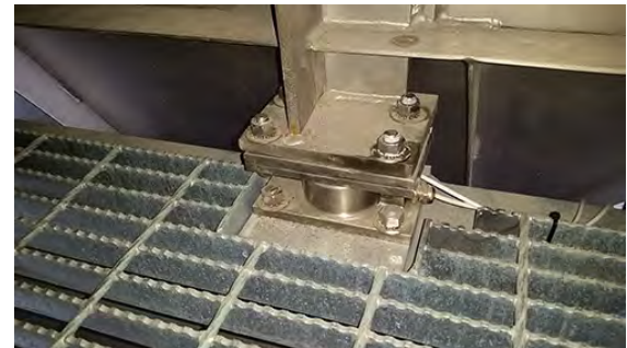
Load Stand Bolts in Place for Easy Installation
