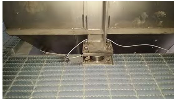
Load Stand is Located Between Vessel and Support Structure
