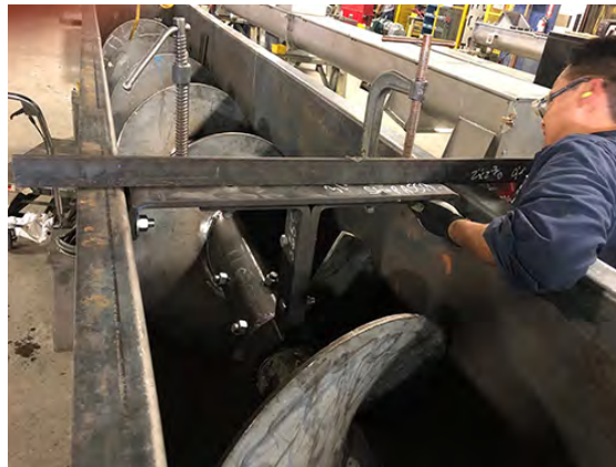
Step 11 – Hanger Bolts are Installed and Tightened to Torque Specifications
