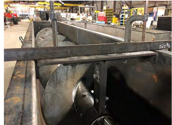
Step 8 – Hanger is Now Flush With Top of Trough
