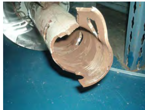
Typical Screw Failure Due to Internal Collar Breaking Free from Pipe
