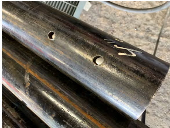
Internal Collar Fits Snugly in Pipe After Holes are Burned
