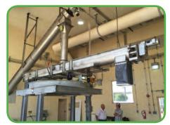
After: New KWS screw conveyor is totally enclosed to contain residuals and odor.
